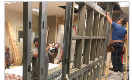
Crews work on the upgraded Salinas Teen Center.
